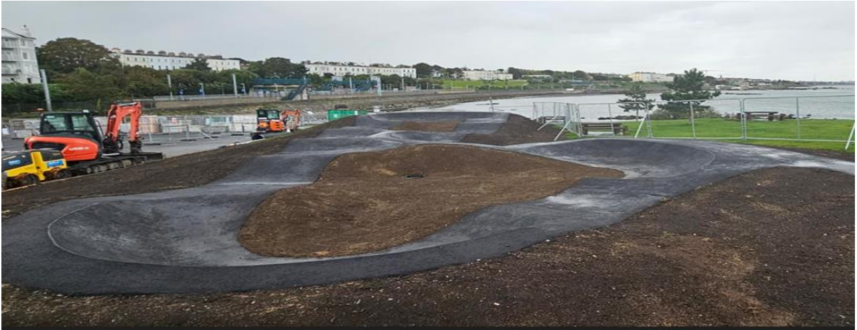
The Pump Track under construction in Apna Park
